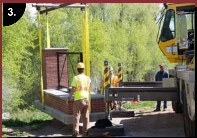
Loading completed base onto trailer
